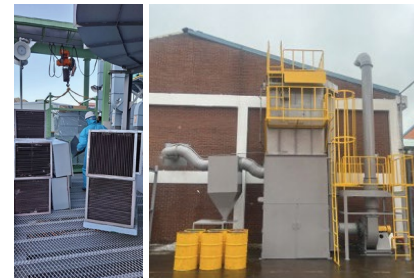
(Left) Filter replacement for bag filter facility (Daedong) (Right) Air pollution prevention facility (Daedong Mobility)
