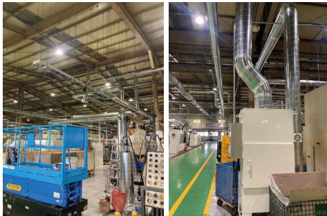
Dust collector installation
