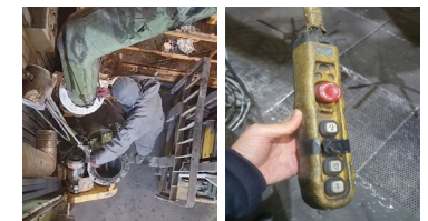
(Left) Dust cleaning inside ducts (Right) Replacement of pendant switch buttons
